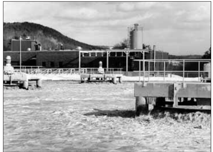
Early 1970s wastewater treatment facility with extended aeration lagoon and platform-mounted mechanical aerators.
