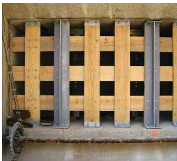
Figure 8. Secondary baffle (SB) type, with 12-inch by 12-inch openings. Krish Ramalingam
