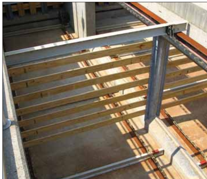
Figure 9. In-tank baffles (In-TB), 8-inch wooden planks evenly spaced at 8 inches. Krish Ramalingam
