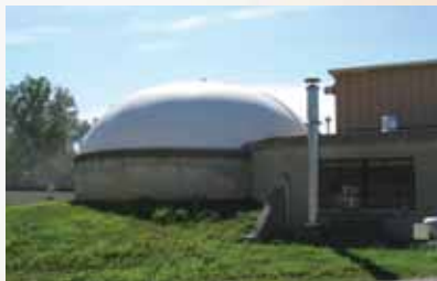
Digester Gas Holding Cover
