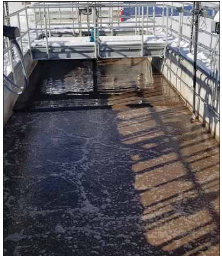
Bioreactors – One of three first stage aerobic zones of BNR system.
