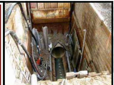
Sliplining of 48" Diameter Interceptor
