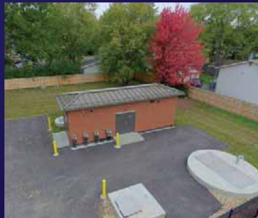
Prefabricated Housed Pumping & Equipment Systems
