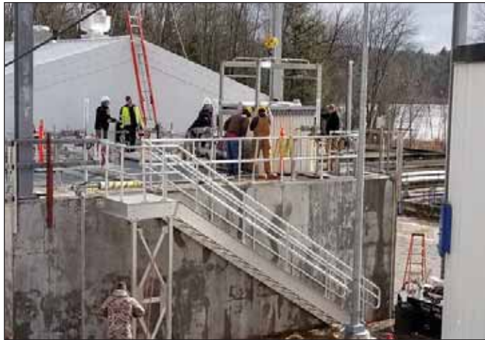
Membranes being installed in the MBR tanks.
