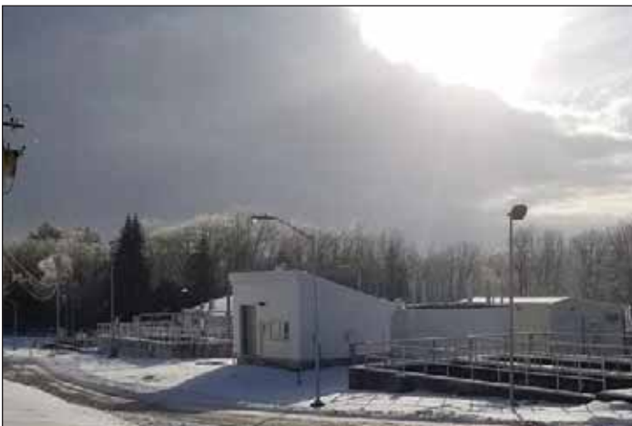
Shot of plant looking from headworks downstream.
