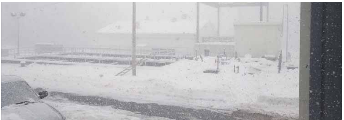
The cold weather brought by the polar vortex in January 2019 posed challenges during start-up operations of the new MBR.
