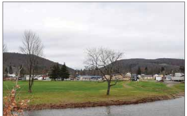
Photograph 2 (after). The completed Walton floodplain project in late 2019.
