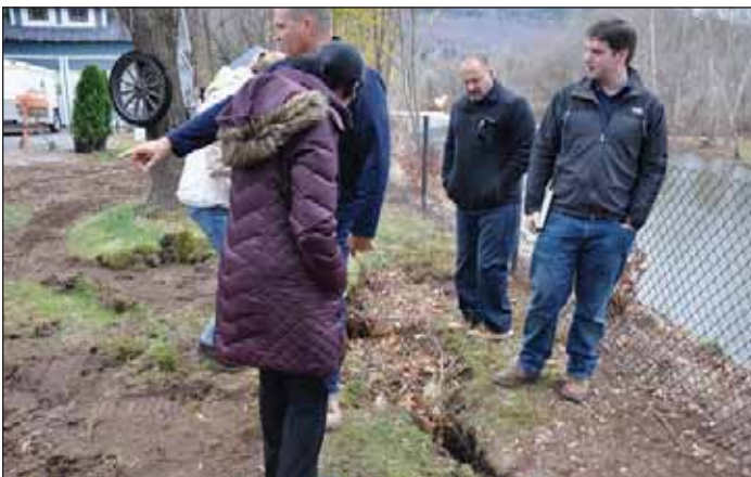
Photograph 4. Graydon Dutcher showing the Army Corps’ Rifat Salim (foreground) and other agency representatives the tension cracks in South Street.
