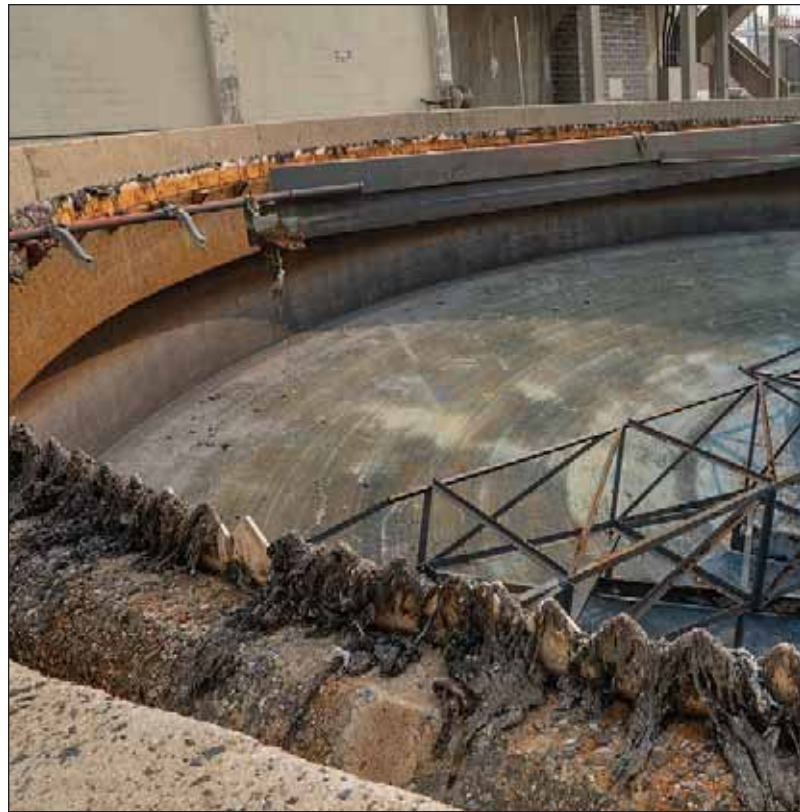
Empty thickener clarifier tank being repaired and cleaned due to wipes damage.
