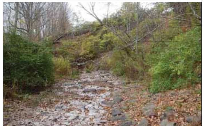
Photograph 6 (before). Hardscrabble’s steep eroding embankment.
