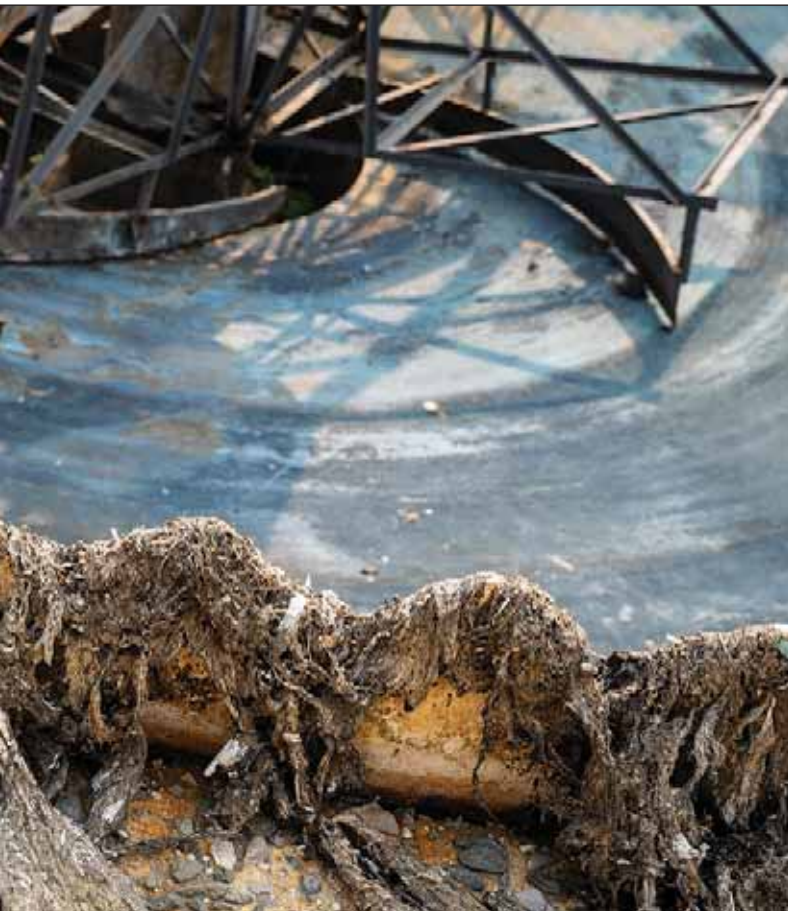
Weir of empty thickener showing rag accumulation. Jean Schwarzwald/DEP
