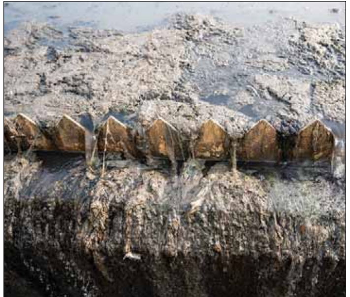
Wipes creating clogs in the thickener clarifiers at Wards Island WRRF. Jean Schwarzwald/DEP
